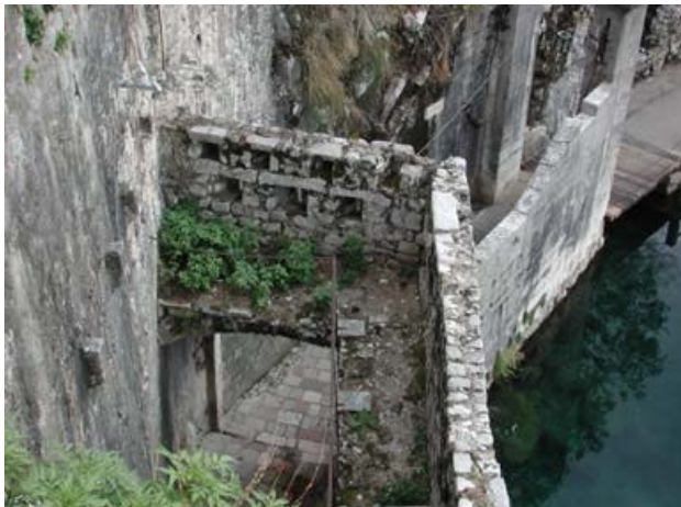
The porch and the walkway from the inside of the fort.
