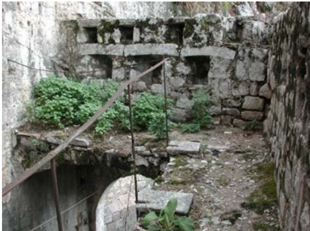
The upper part of the walkway.
