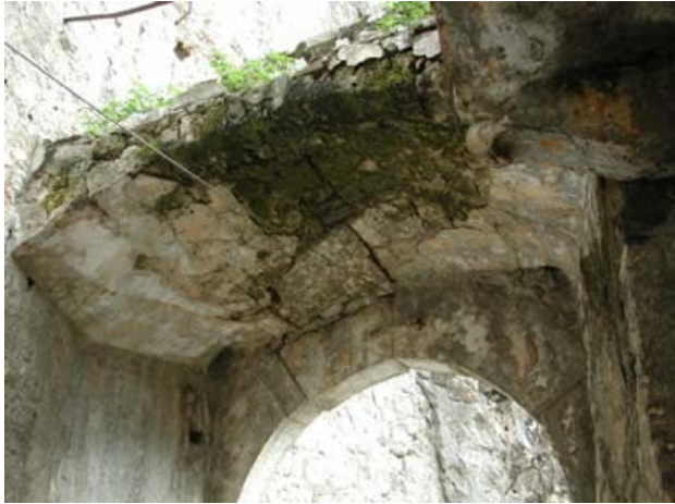
The under-side of the porch.
