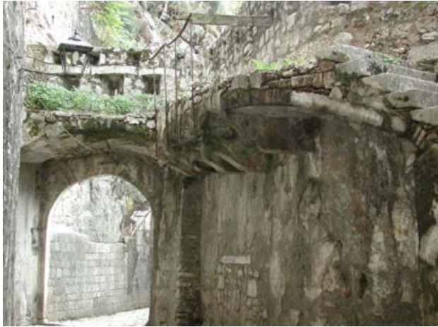
The hanging walkway.
