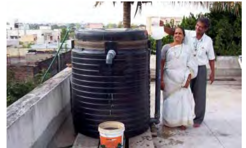
Example of household size biogas plant
