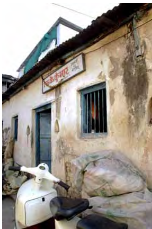
Thick adobe walls are typical of the small scale houses in Kumbhar Wada.
