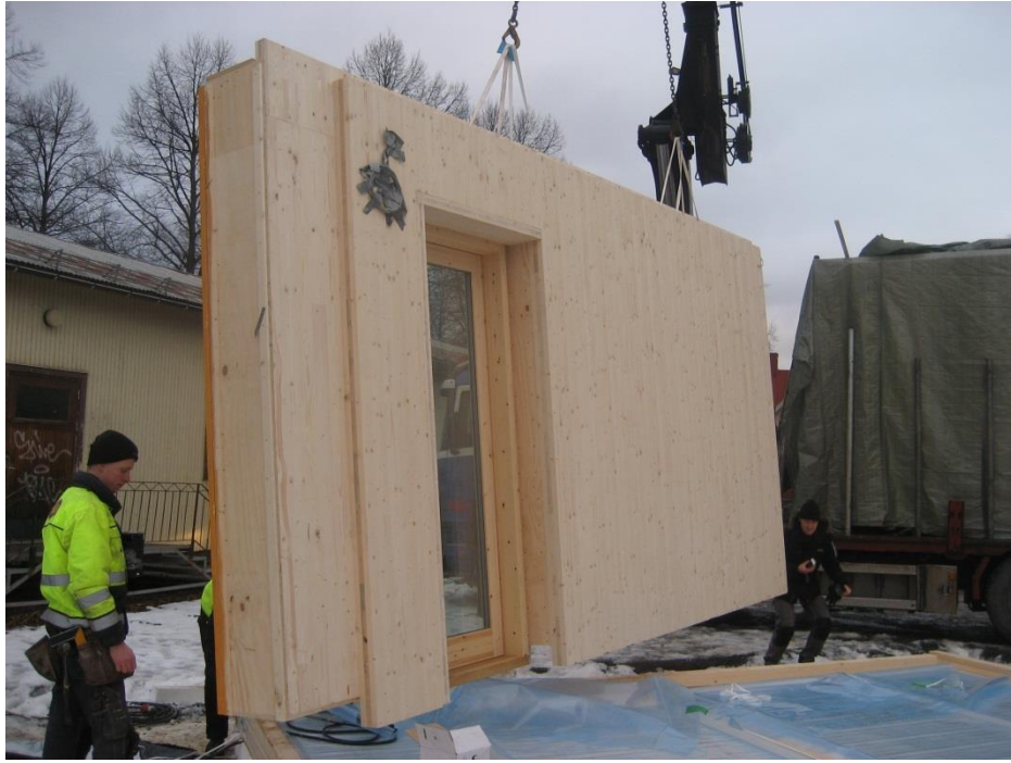
Figure 14. Assembly of the north wall. The position of the lifting loops means that the wall leans somewhat which makes placing it on the floor element more difficult.
