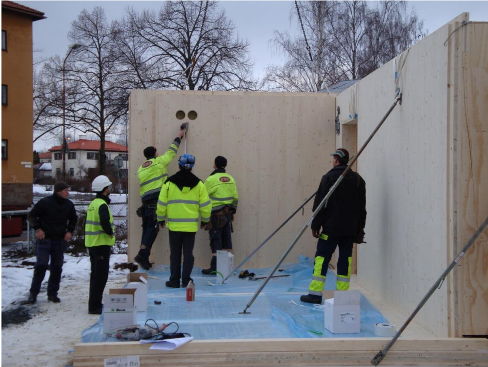
Figure 16. Assembly of the west wall.
