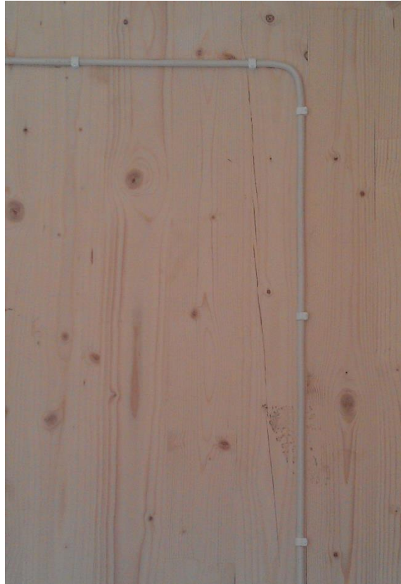
Figure 12. The picture shows cracking in a CLT panel approx. five months after the assembly of the building. However, thermography in connection with pressure testing shows no sign of this cracking causing any extra air leakage, partly because the CLT panel is built up of several layers.
